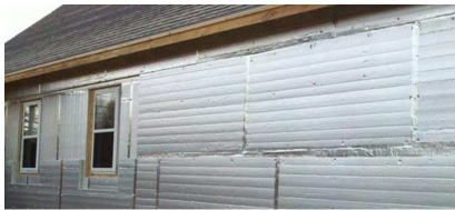
Two layers of 2" rigid insulation on exterior for energy reduction. Ceiling: cellulose+2" expanding foam (R-80)
